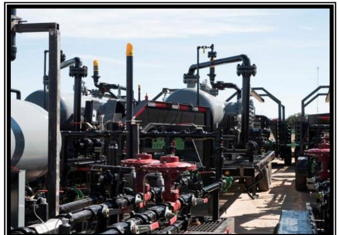
A multi package project consisting of three phase separator, vertical low pressure separators, monorails, sand separators and four phase separators
